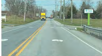
Existing traffic spacing markings
