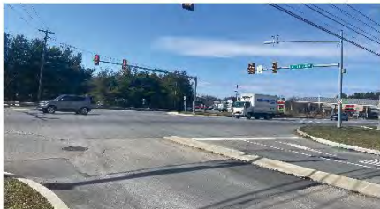
Wide crossings with no crosswalks or pedestrian facilities
